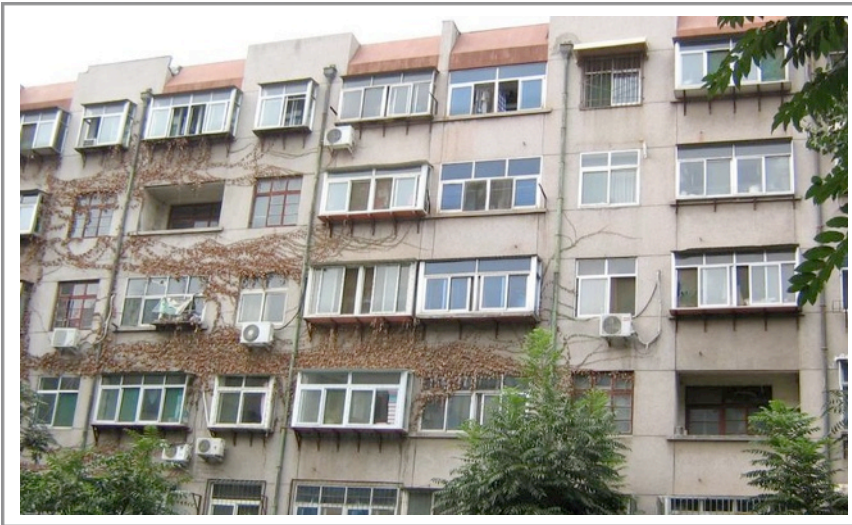
Figure 27: Welfare Apartment Building
