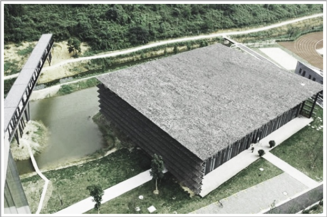
Figure 10: Bridge of China Academy of Art
